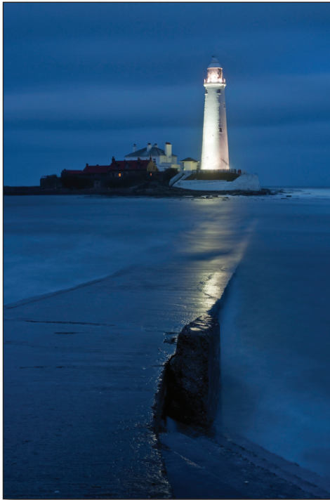
St Mary's Lighthouse, near Whitley Bay, which was completed in 1898 and remained in operation until 1984. A causeway, accessible only at low tide, allows visitors to reach the island on which the lighthouse sits.
